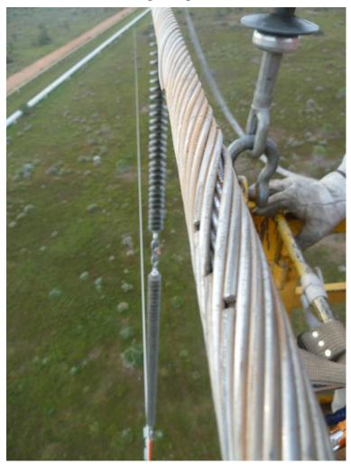
Figure 2 - Transmission Line Conductor showing damaged strands
