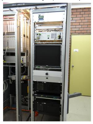
Figure 2 SVC 2 secondary system cabinet including computer control system.
