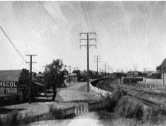
THE NUMBER 4 LINE FROM OSBORNE, SHOWN HERE FROM THE RAILWAY BRIDGE AT ETHELTON, USED THE NEWLY DESIGNED STOBIE POLE IN ITS CONSTRUCTION. THE STOBIE POLE WAS OF ENORMOUS SIGNIFICANCE TO THE PACE AT WHICH AESCO'S SYSTEM SPREAD ETSA MUSEUM
