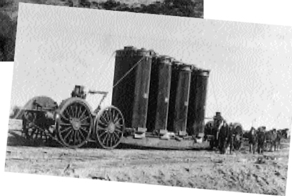
A VIEW OF OSBORNE “A” POWER STATION, 1924, FROM THE WEST AND, DURING THE CONSTRUCTION OF THE POWER STATION, ON 21 MAY 1923, THE HAULING OF MASSIVE TRANSFORMERS ON A CROCODILE TRUCK BY HORSEPOWER ELECTRA.NET SA, ETSA MUSEUM
