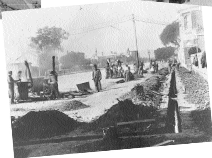
LAYING ELECTRICAL TRANSMISSION LINES UNDERGROUND IN ADELAIDE, 1901–1902, STRETCHING FROM GRENFELL STREET POWERHOUSE, TO WAKEFIELD STREET, TO VICTORIA SQUARE – PASSERSBY AND TRADERS TAKE IN THE SCENE OF LABOURERS STRIVING WITH PICKS AND SHOVELS. THE WAKEFIELD STREET SCENE ALSO SHOWS BOILERS CONTAINING HOT BITUMEN – THE PITCH WAS USED FOR SEALING JOINTS IN THE CABLES AND CABLE HOUSING ETSA MUSEUM
