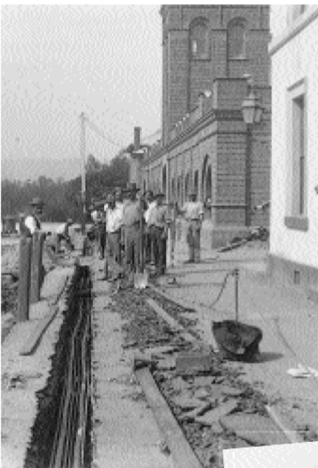
LAYING ELECTRICAL TRANSMISSION LINES UNDERGROUND IN ADELAIDE, 1901–1902, STRETCHING FROM GRENFELL STREET POWERHOUSE, TO WAKEFIELD STREET, TO VICTORIA SQUARE – PASSERSBY AND TRADERS TAKE IN THE SCENE OF LABOURERS STRIVING WITH PICKS AND SHOVELS. THE WAKEFIELD STREET SCENE ALSO SHOWS BOILERS CONTAINING HOT BITUMEN – THE PITCH WAS USED FOR SEALING JOINTS IN THE CABLES AND CABLE HOUSING ETSA MUSEUM
