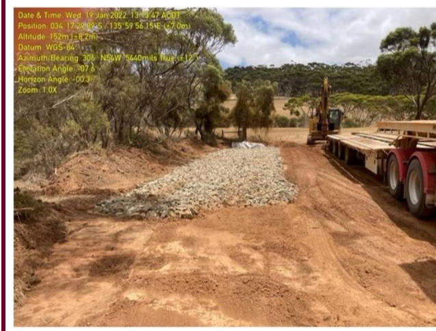
Structure 648 Washdown Bay
