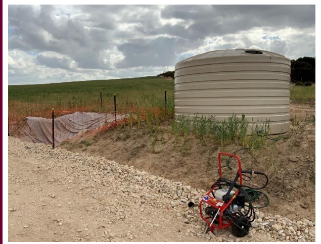
Structure 167 Washdown Bay
