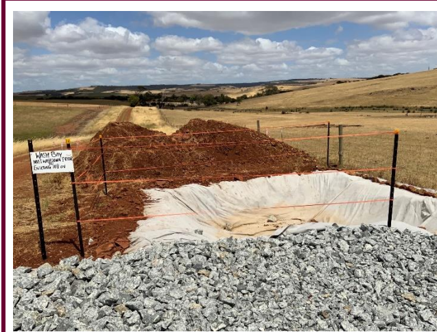
Structure 708 Washdown Bay
