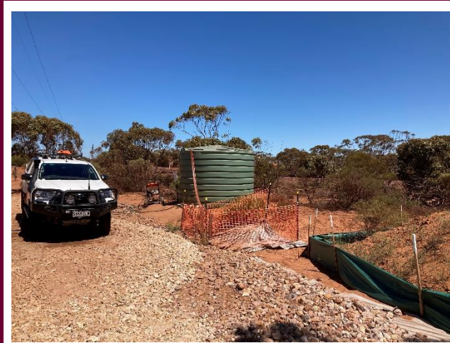
Structure 84 Washdown Bay
