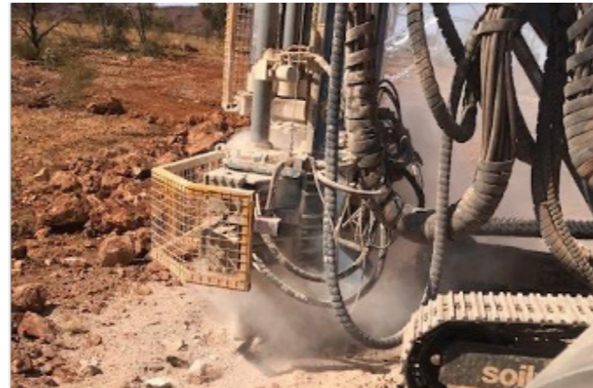
Drilling foundations
