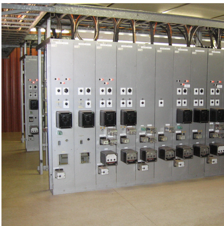
Figure 2 - Protection relays at Davenport substation
