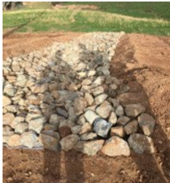
Rock and geotextile
