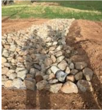
Rock and geotextile
