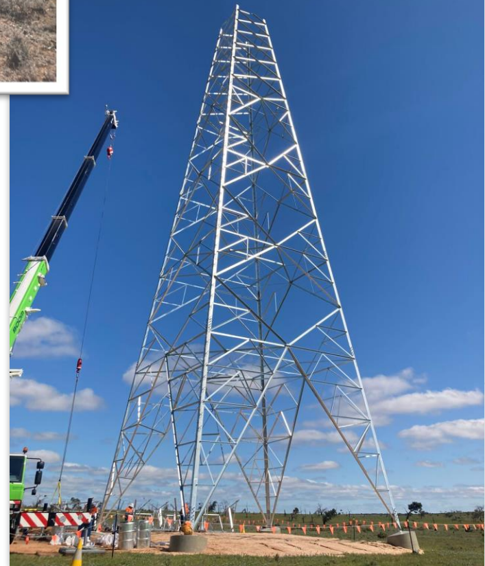
Erection of first 330 kV tower in SA
