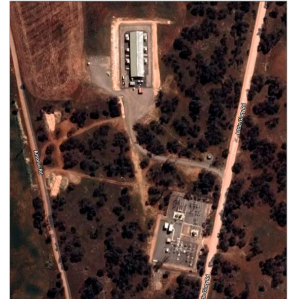
BESS and Dalrymple substation
