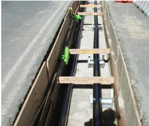
Figure 4-16 Typical Cable Trench in Concrete Roadways
