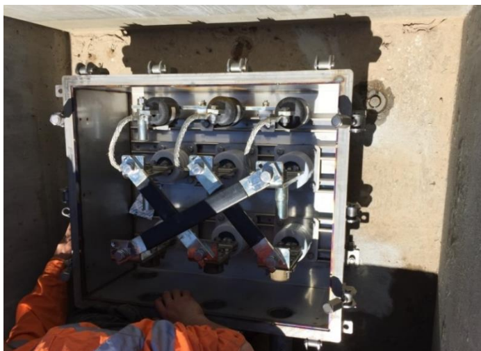
Figure 4-9 Typical Arrangement of Link-Box in Underground Concrete Pit
