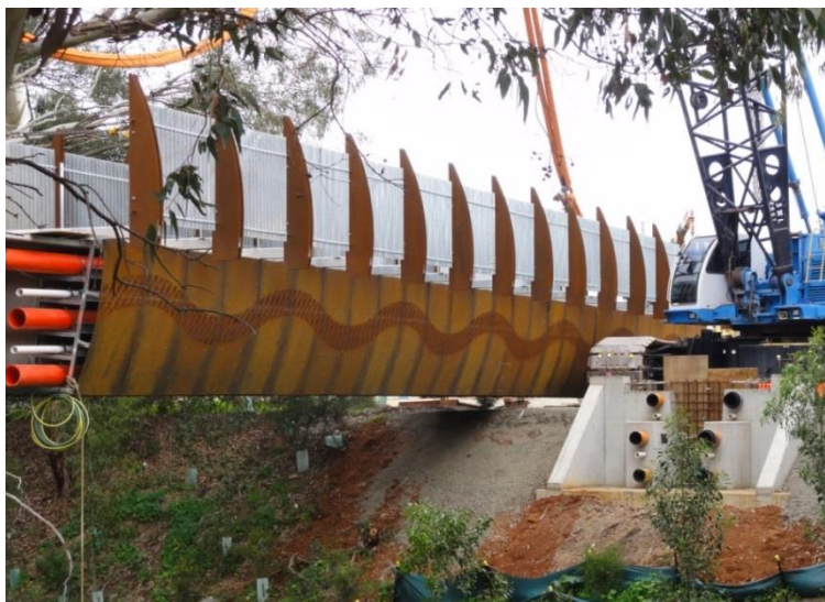
Figure 4-21 Typical Purpose-Built Cable Bridge Construction
