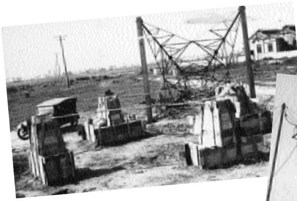
THE CROSSING OF THE PORT RIVER BY TRANSMISSION LINES WAS A DIFFICULT TASK. IN AUGUST 1924, TOWERS SUCH AS THIS ONE WERE ERECTED. THE SPAN BETWEEN TOWERS WAS ABOUT 300 METRES ETSA MUSEUM
