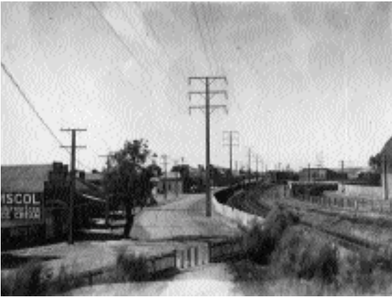
THE NUMBER 4 LINE FROM OSBORNE, SHOWN HERE FROM THE RAILWAY BRIDGE AT ETHELTON, USED THE NEWLY DESIGNED STOBIE POLE IN ITS CONSTRUCTION. THE STOBIE POLE WAS OF ENORMOUS SIGNIFICANCE TO THE PACE AT WHICH AESCO'S SYSTEM SPREAD ETSA MUSEUM
